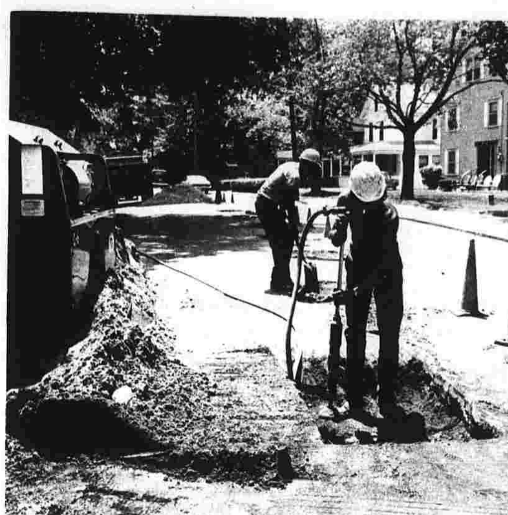
Gas main repair work under way
